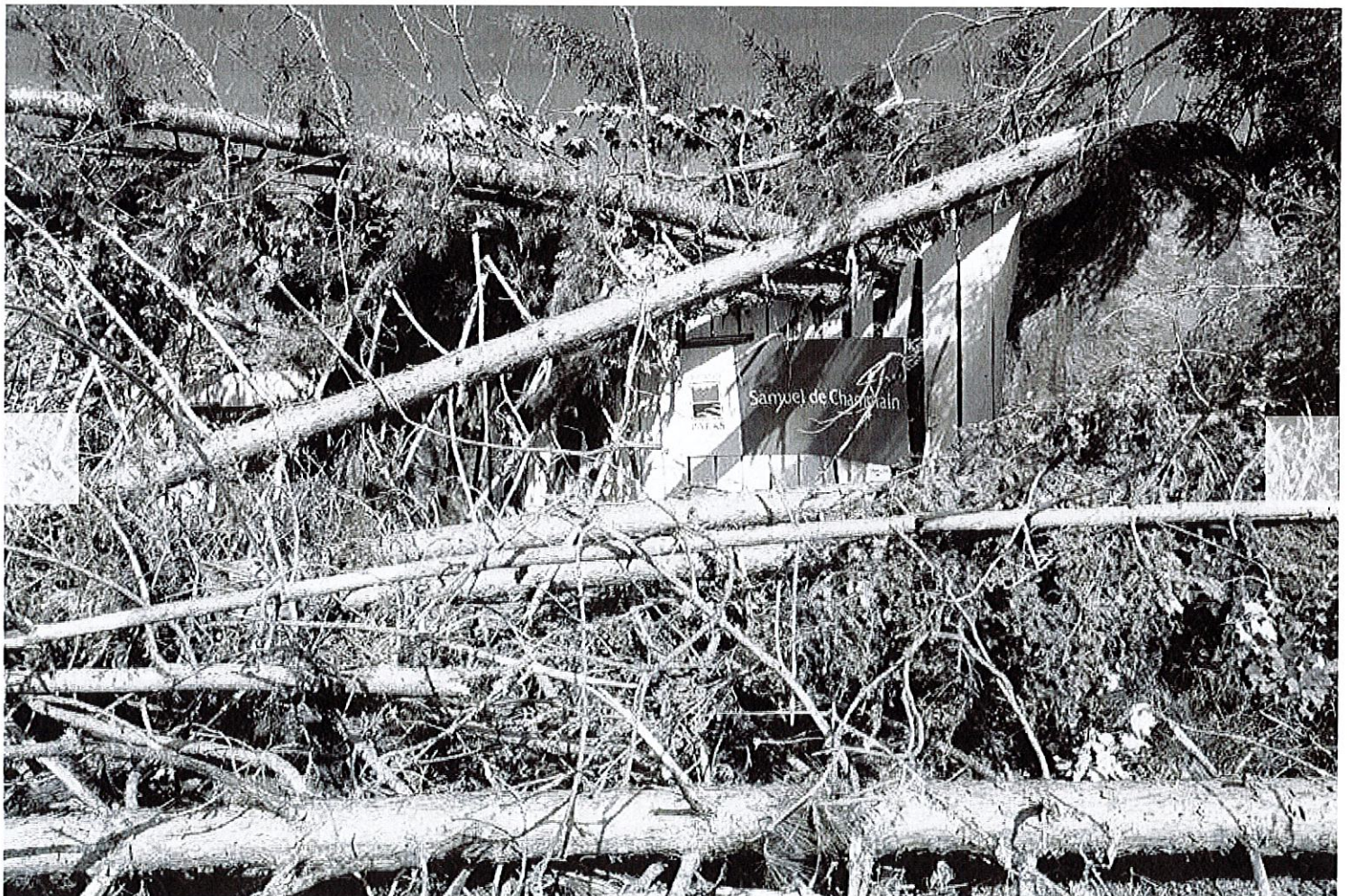
1 / 3 After the storm hit on July 21, 2025, trees covered the entrance to Samuel de Champlain Provincial Park. Mayor Gould and Calvin Township's council are reminding the province that much of the township still has thousands of fallen trees, and need help cleaning up. / File | Photo by David Briggs
